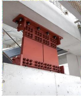
Figure 1. Viscoelastic Damper (VED) Panels
