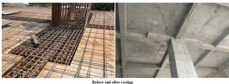
Figure 1. Construction retrofitting beam on apartment in Yogyakarta
