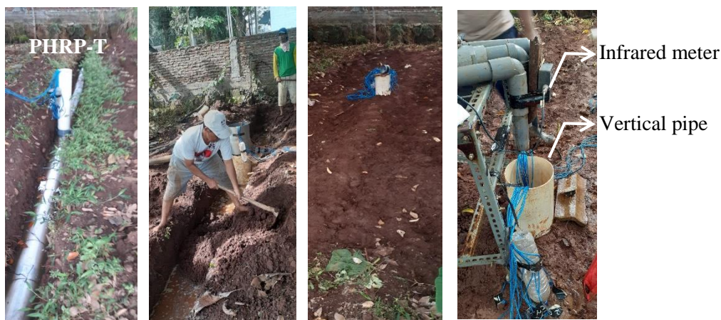
Figure 2. Assembly and installation of PHRP-T for testing
