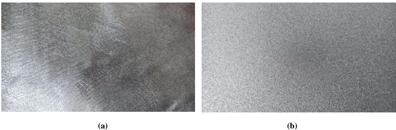
Figure 4. Visual After Surface Preparation: (a) power tool cleaning, (b) abrasive blast cleaning
