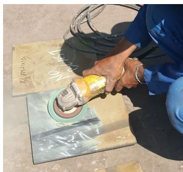
Figure 1. Surface preparation with a power tool
