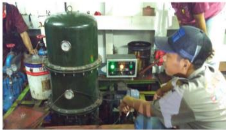
Gambar 2. Commissioning OWS System
