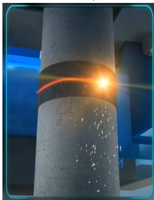
Gambar 7. Ilustrasi Penyambungan Tiang Pancang (Jack Xie (T-Works), 2013)
