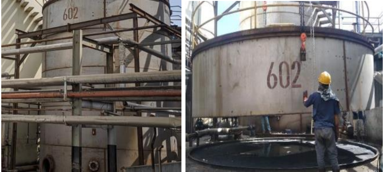
Gambar 4. Realisasi Alat Tank Erection Manual Jacks
