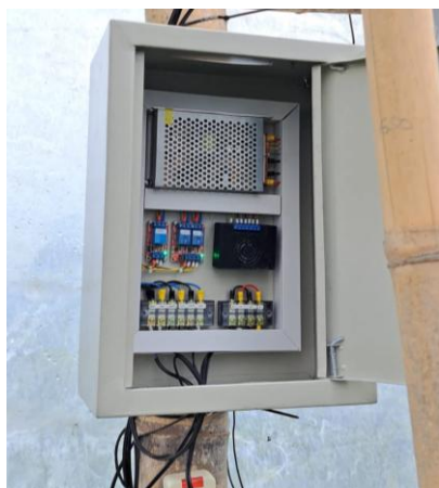
Fig 8. ChrysoSmart control panel installed in the greenhouse for actuator control
