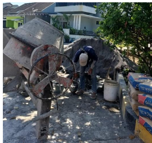
Gambar 3. Proses Mixing Mortar Pasangan batu
