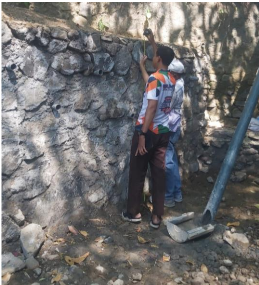
Gambar 5. Proses Finishing Dinding Penahan Tanah
