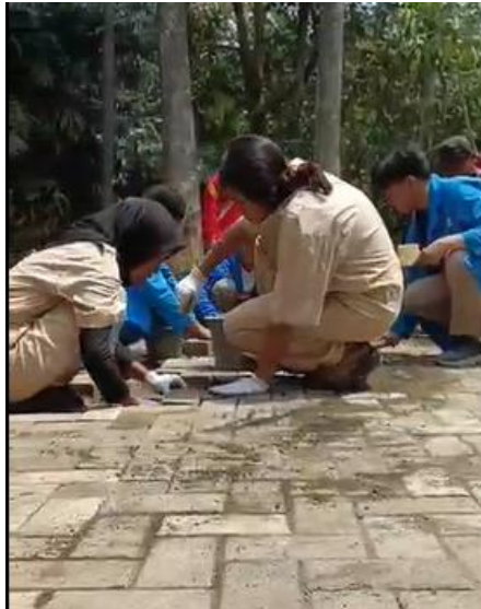
Gambar 5. Pengisian Nat Paving Block
